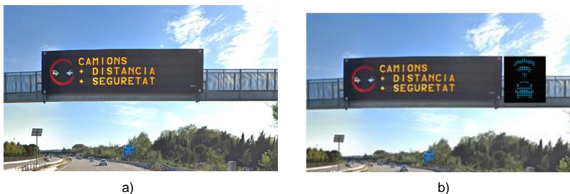
Figure 3 – PK 62,28: a) VMS with a pictogram on the left and three lines of text b) VMS plus full-color pictogram added for the project
