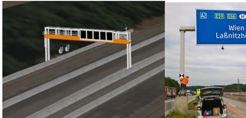
Figure 4 – Gantries equipped with ADAS
