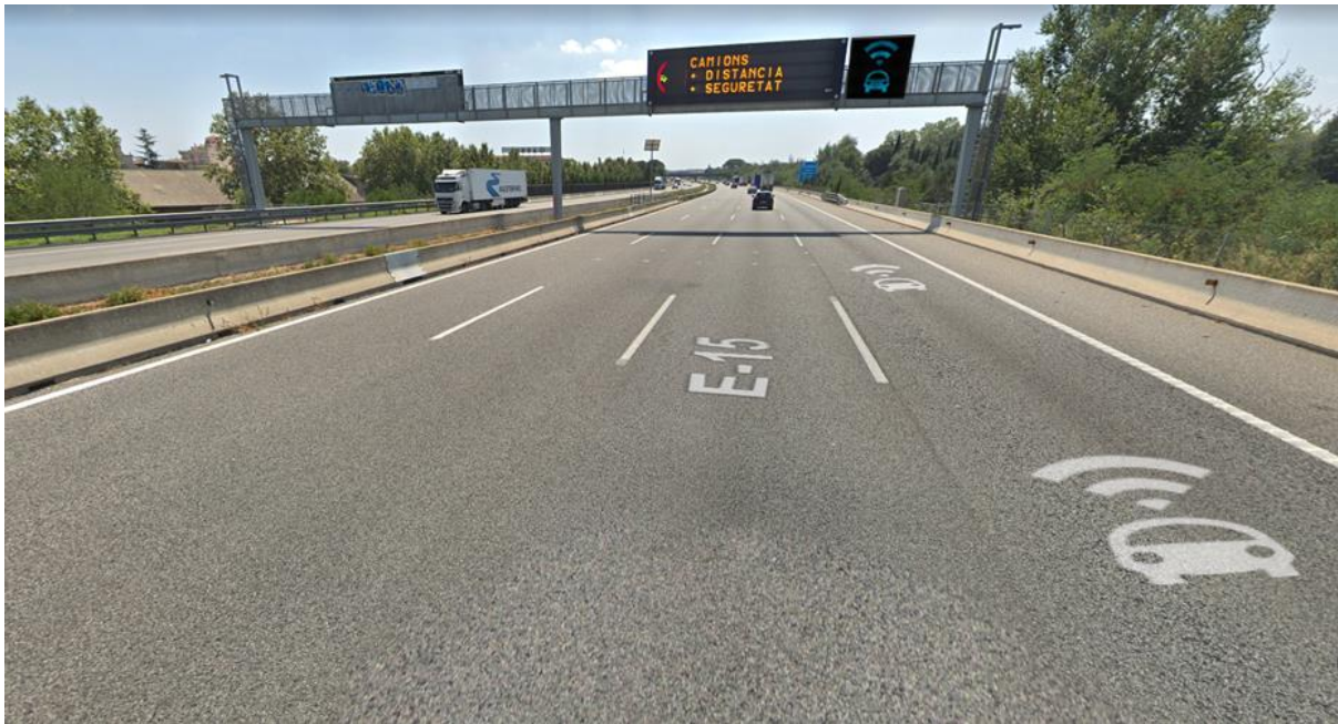
Figure 38 – New sign on asphalt and gantries VMS, final design
